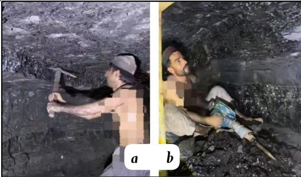
Figure 8 (a & b) Workers working with no PPE pictures was taking during data collection
