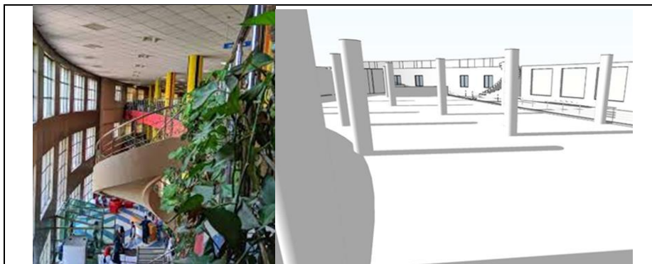
Figure 12:(a) Atrium at the time of electric breakdown,(b) depth of shadows at 4:00pm from the South.
