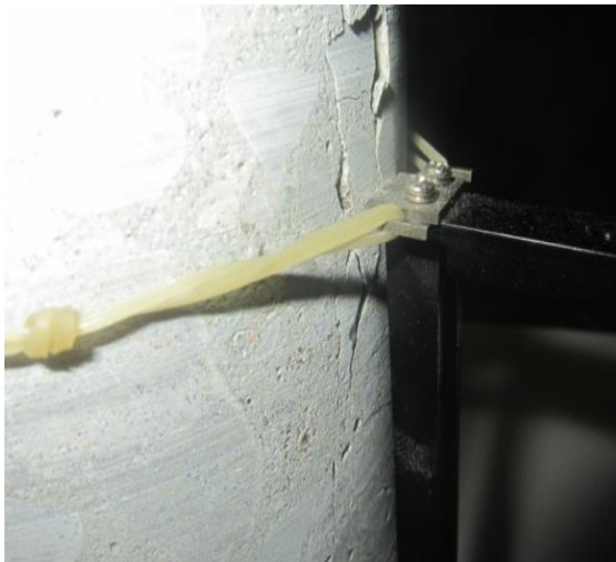
Fig. 9 - OLD1 Specimen crack propagation
